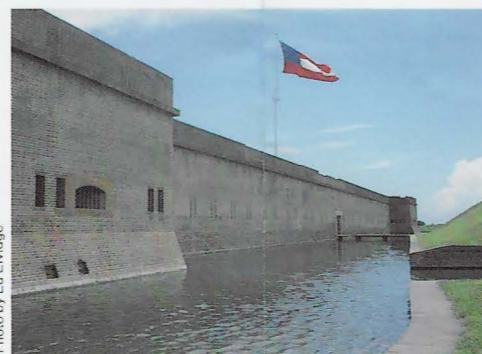
This view along Pulaski's exterior gorge wall shows part of the moat and the fort's entrance and drawbridge.
