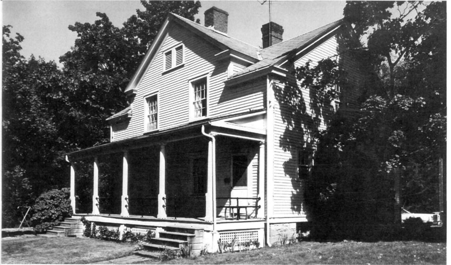
Double non-commissioned officers' quarters, southwestern elevation.
