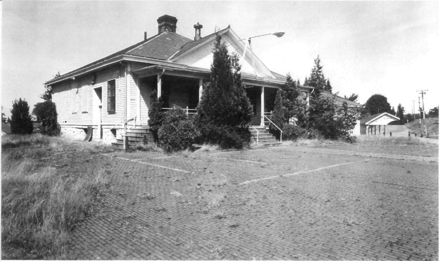
Guard house, southern elevation.
