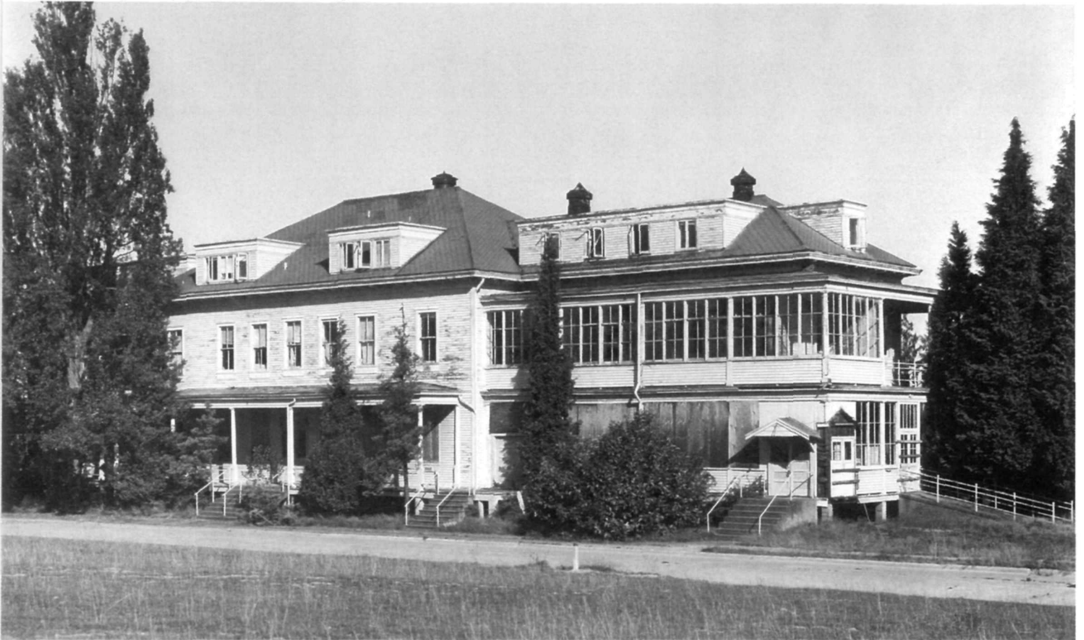
Hospital, one of the earliest buildings completed on the post.
