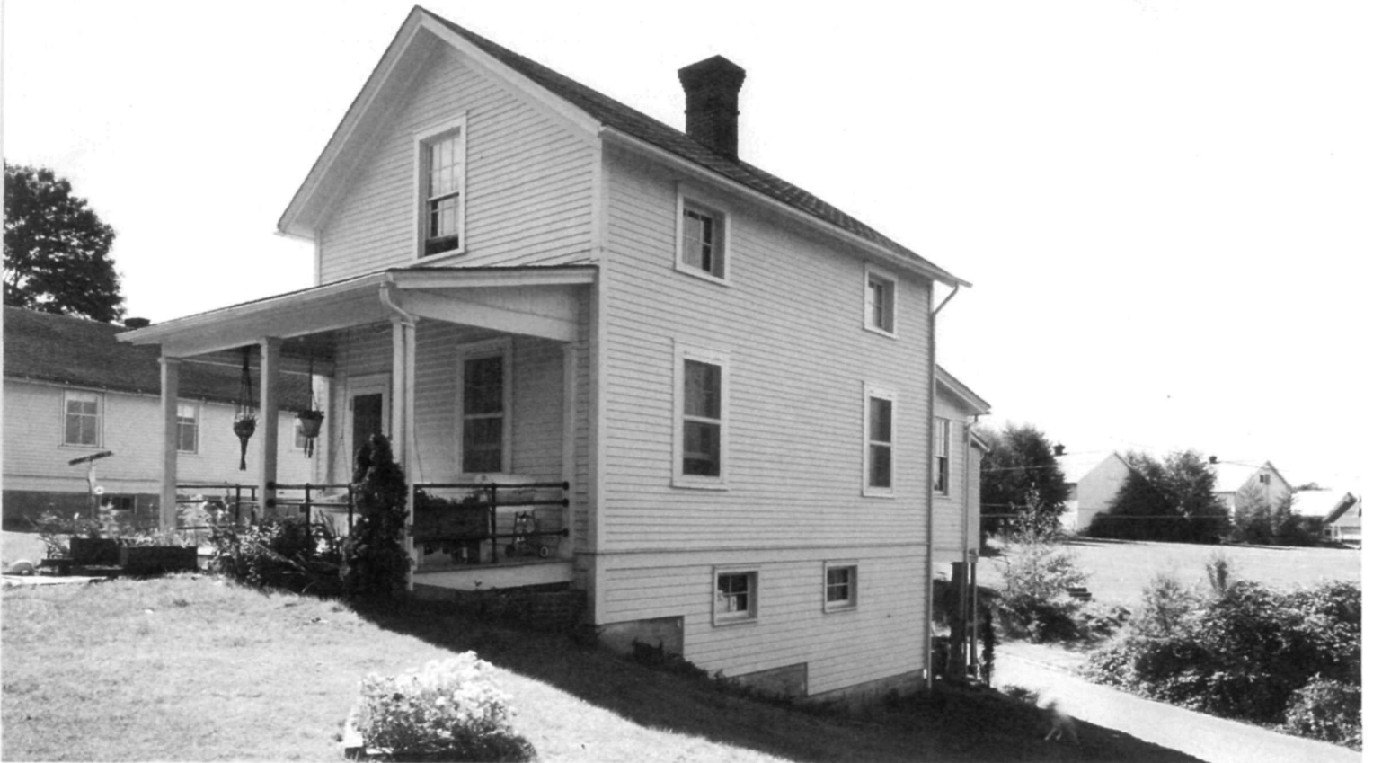
Hospital steward's quarters, northeastern elevation.
