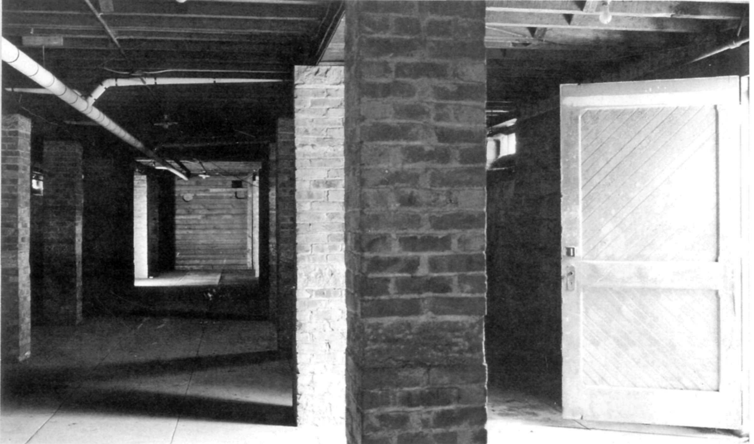
Quartermaster storehouse—basement brick piers.
