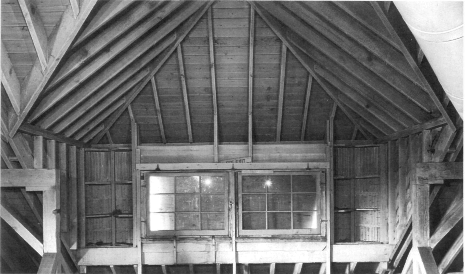
Double barracks attic—detail of dormer framing.
