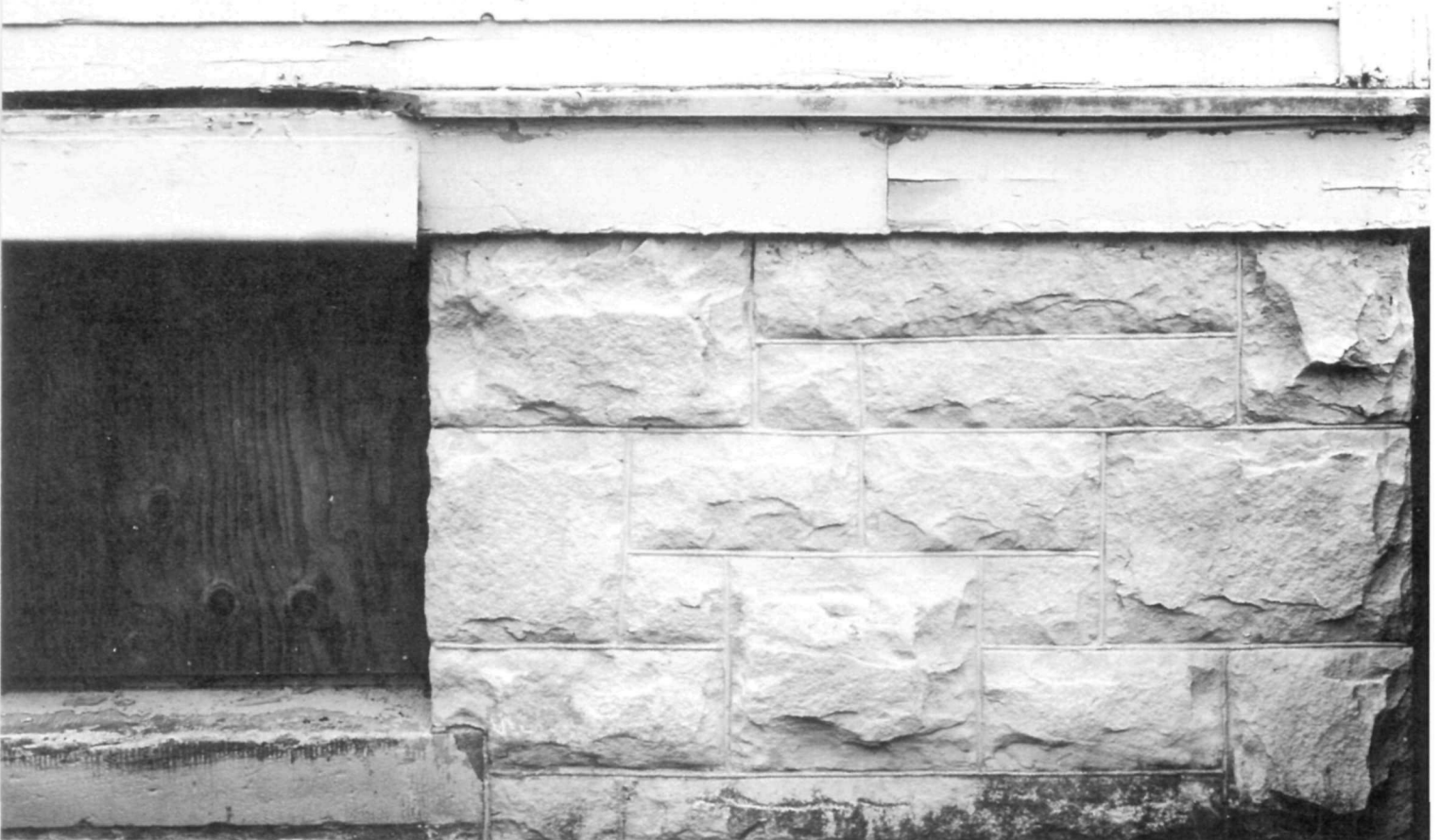
Double barracks—detail of sandstone foundation.
