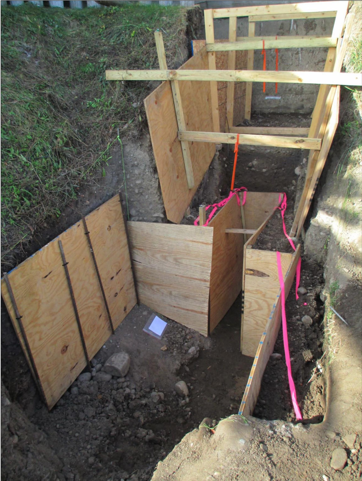
Figure 32: 2013 Trench Stabilized Prior to Backfill
