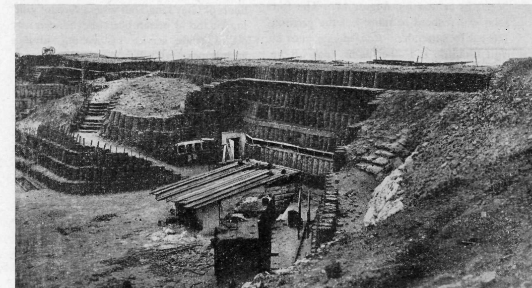
The Confederate defenders converted the masonry fort into an earthwork during the siege of 1863-64.
