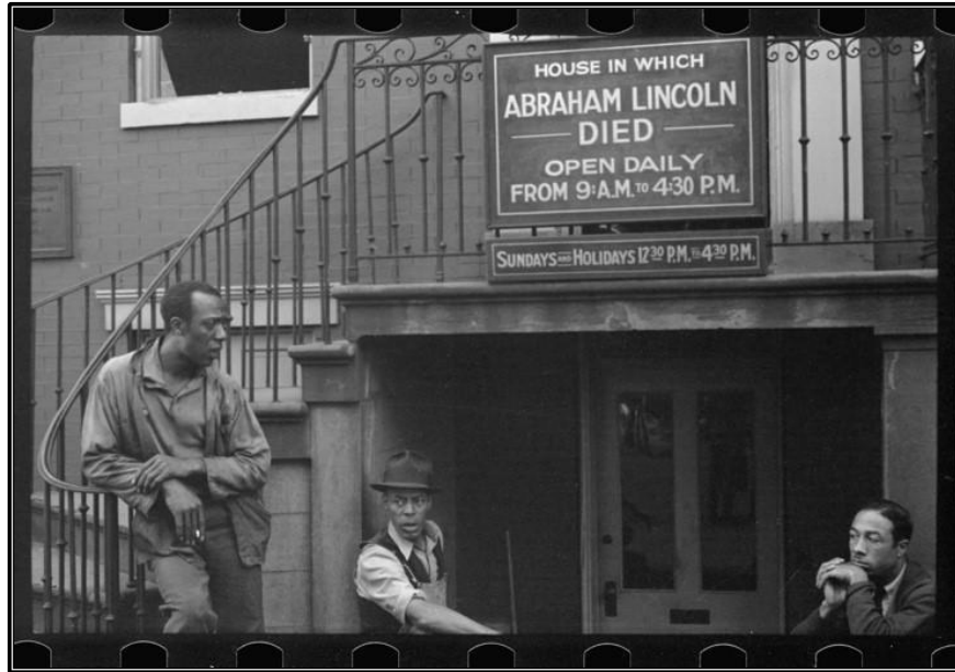
Figure 2.6. House Where Lincoln Died, showing pre-NPS sign, December 1937. (Photo by John Vachon. Washington, D.C. House Where Lincoln Died , Farm Security Administration - Office of War Information Photograph Collection, Prints and Photographs Division, LOC.)
