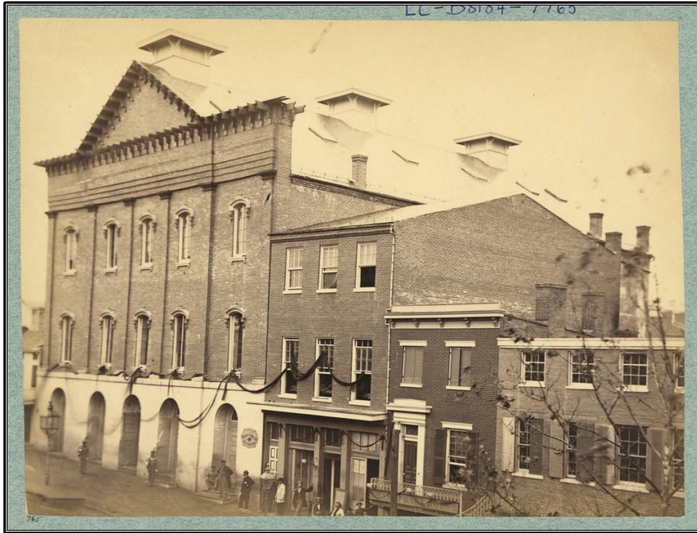
Figure 1.3. Ford's New Theatre, ca. 1865. This photograph was taken following the assassination and shows clearly the unfinished cornice and other details of the building. The Star Saloon is visible to the immediate right of the theater ( Ford's Theatre, scene of the assassination . Prints and Photographs Division, LOC).
