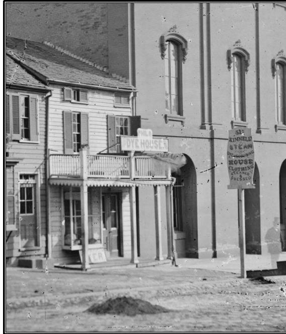
Figure 5.1. Detail of Ford's Theatre photograph, showing 517 Tenth Street, NW, then a two-and-one-half-story frame building housing Kimmell's Dye House, ca. 1872 ( Ford's Theatre, Wash. D.C. , Brady-Handy Photograph Collection, Prints and Photographs Division, LOC).
