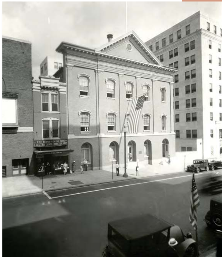
1931 exterior of Ford's Theatre. Note: To the right of the theatre the Star Saloon building has been removed and the area used for parking. See picture on page 4 for comparison. (NPS collection)
