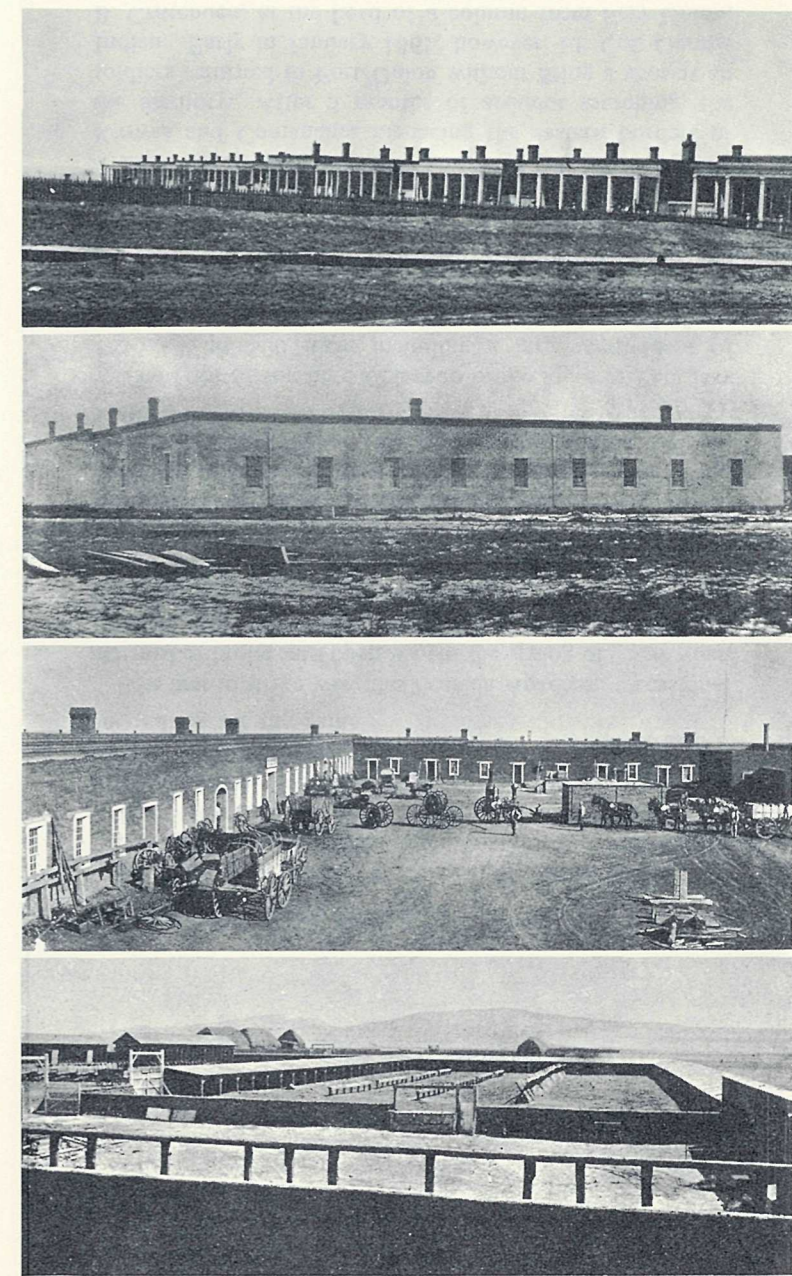
The third and last fort was almost a city in itself. Erected between 1863 and 1869, it consisted of the post of Fort Union and the Fort Union Quartermaster Depot. Above are officers' quarters and barracks of the post, below the mechanics' and herders' corrals of the depot.
