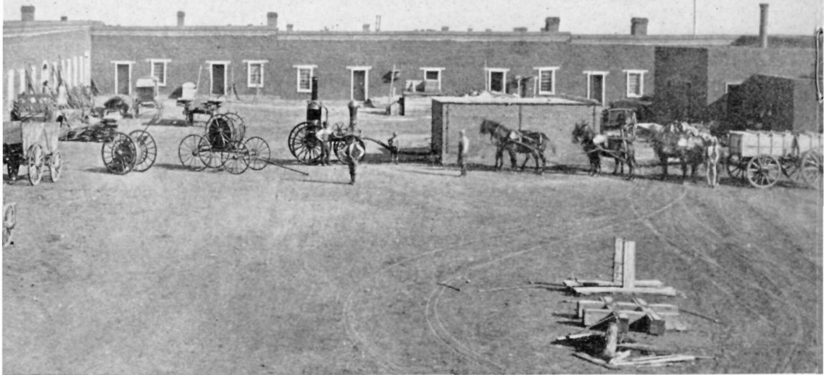
Water tank site—1876.
