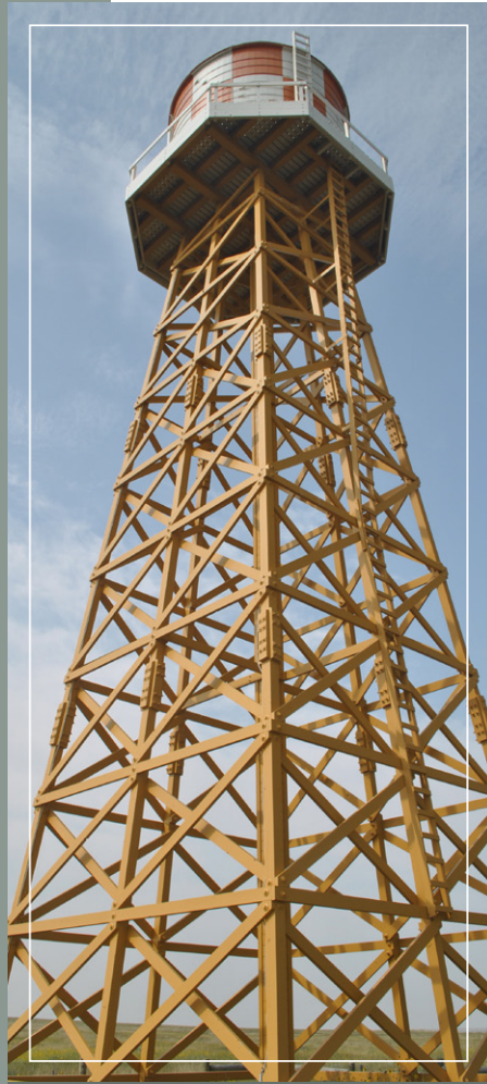
The 72-foot water tower at Amache was reconstructed using some original materials. NPS photo.
