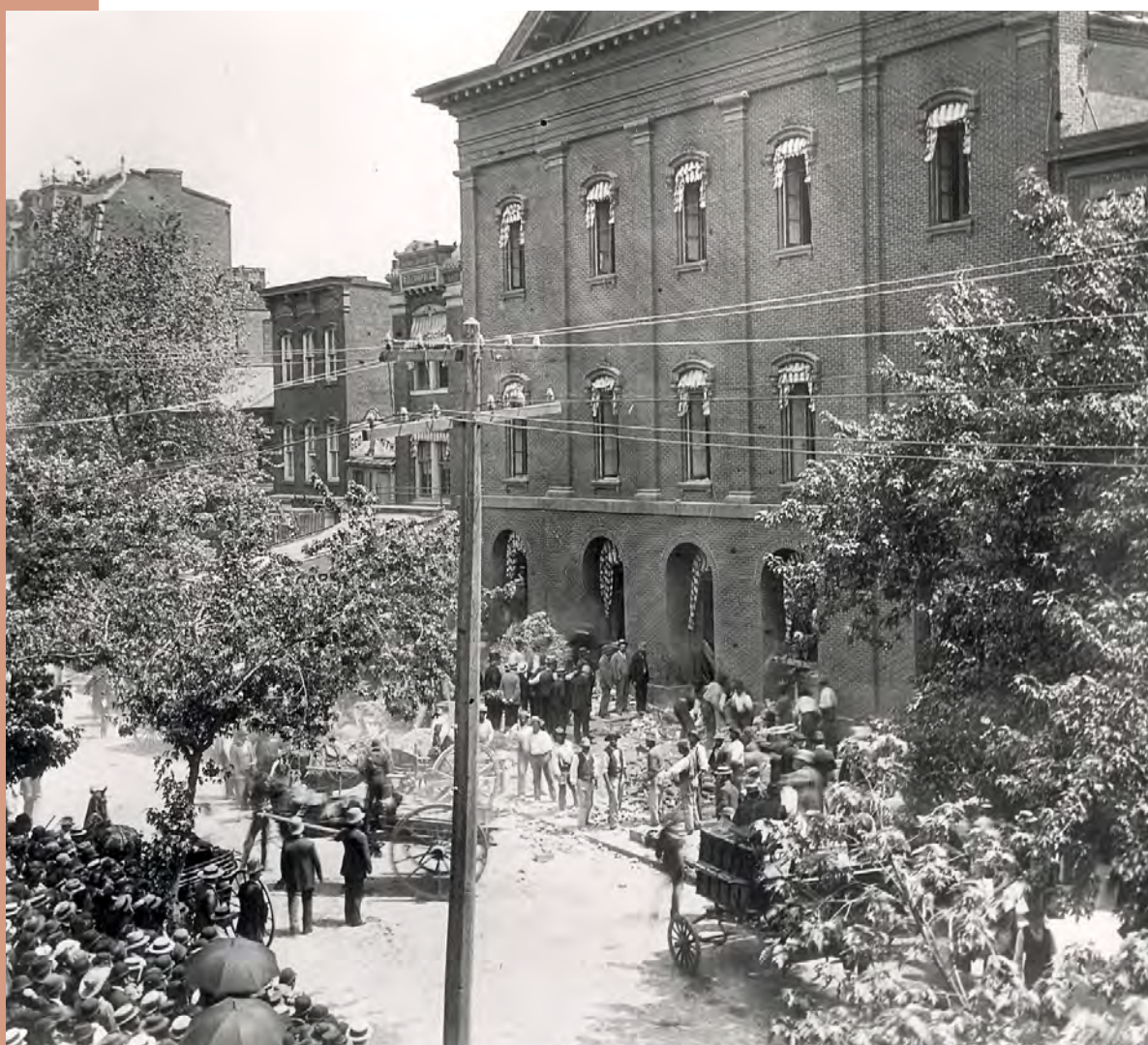
1893 photograph showing crowds gathered outside Ford’s Theatre after collapse of building interior – 22 federal employees were killed and more than 60 were injured. (NPS Collection)
