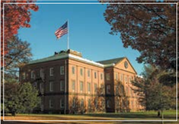
Built in the mid-19th century for storage and maintenance of weapons, this building holds the visitor center, museum, collection, and staff offices.
