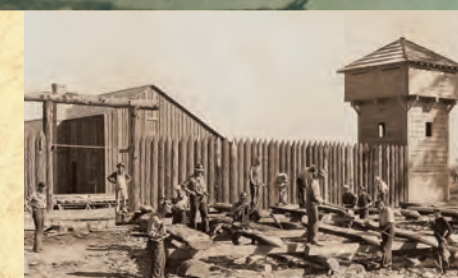
The sales shop, front palisade, or wall, and bastion, at right, are essentially complete in this photograph from September 1, 1934. The work underway in the foreground is the squaring and shaping of additional pickets for the remaining three sides of the palisade that surrounded the reconstructed historic site. Fort Nisqually's original site was 15 miles south, near DuPont.
