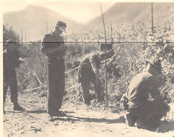
Marshall was very interested in the possibilities presented by the Civilian Conservation Corps, encouraging education "to prepare a boy for a job in civil life, which is the real purpose of the CCC." In this 1930s photo a crew is surveying a road. Courtesy of the National Park Service.
