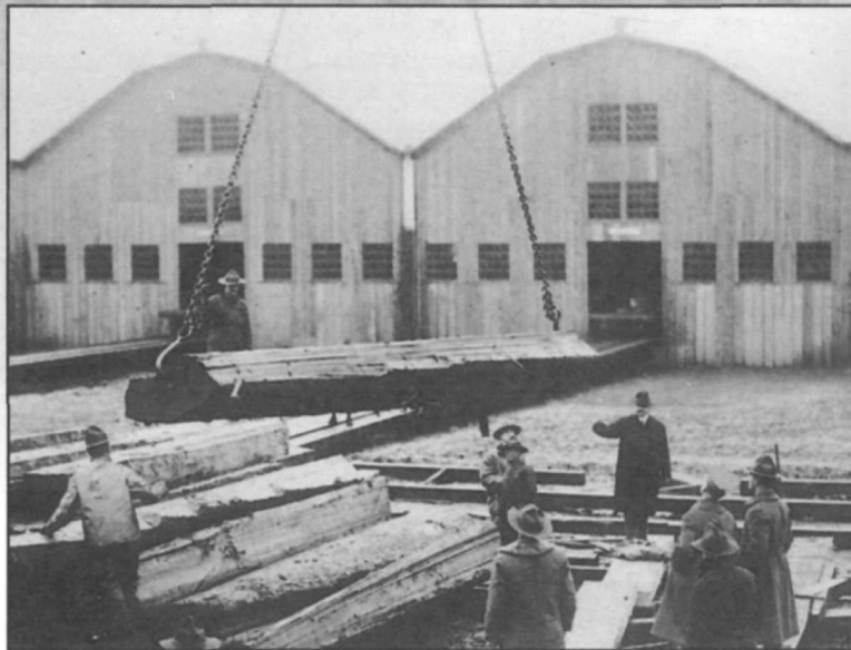
The photo shows a crane unloading a piece of spruce. It will be placed on a stack or “deck,” and then moved into one of the six mill entries. At each entry, there were two huge saws that cut the spruce into smaller planks that were in turn cut into aircraft-size boards. Signal Corps
