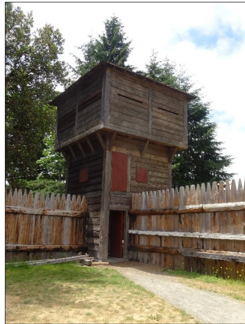
Figure 11. Southwest bastion, June 2019. Photo by the author.
