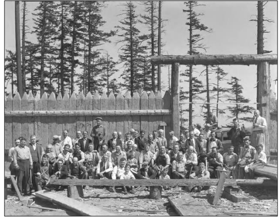
Figure 10. Construction crew in front of palisade, 1934. Tacoma Public Library, Richards Studio no. 804-4.
