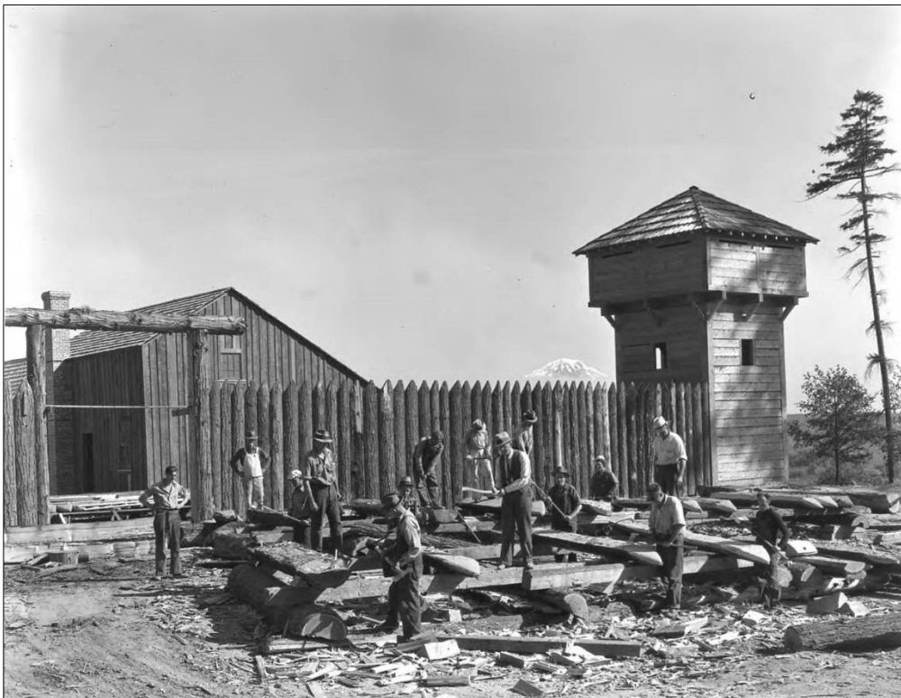
Figure 1. Construction crew working outside the palisade at Fort Nisqually. To the right is the southwest bastion, to the left and through the entrance is the store, and an artistically inserted Mount Rainier peeks over the palisade in the center. Photograph taken September 1, 1934. Source: Richards Studio 804-6, Tacoma Public Library Digital Collections. [Fort Nisqually Living History Museum has the original photo, sans mountain.]
