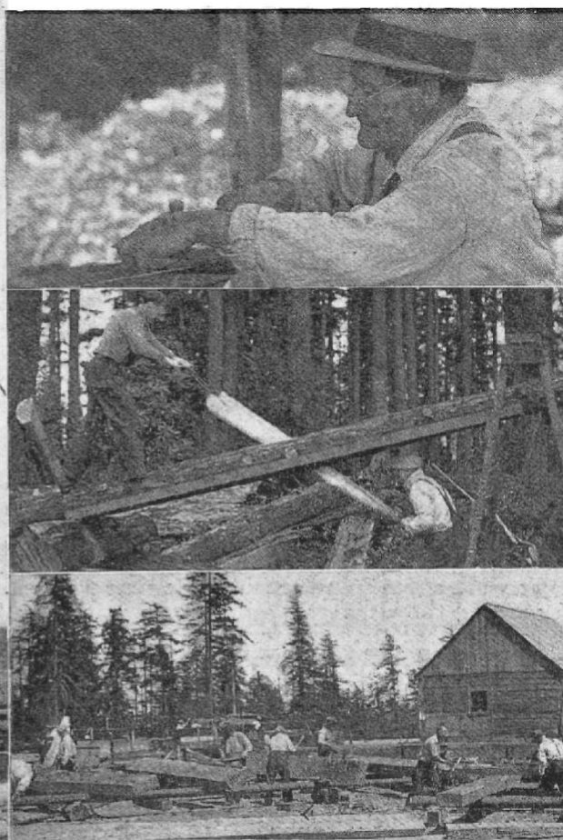
Lower left: The bastion goes up. Below: Saw filer truing a whip-saw; Whip-sawing planks—old style; Squaring logs in the timber yard.
