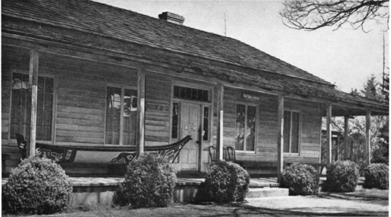
When Fort Nisqually was reconstructed at Tacoma overlooking Puget Sound, 15 miles from the original site, the Factor's house of 1854 was one of the two old buildings restored.
