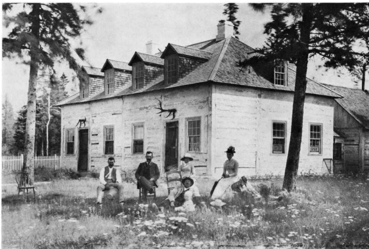
The Company house built at the end of the Grand Rapids Tramway in Central Manitoba was an example of 'Red River frame' or posts on the sill construction. Photograph by J.B. Tyrrell, 1890.
