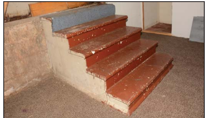
Figure 32: Non-contributing concrete stairs located at the rear of the warehouse space.
