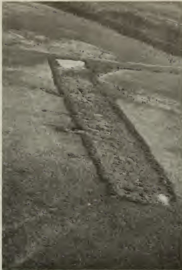
Illustration 5. Unusable airstrip constructed in moist tundra near Mascot Creek. Note ponding of water and vegetational changes caused by thawing of underlying permafrost.
