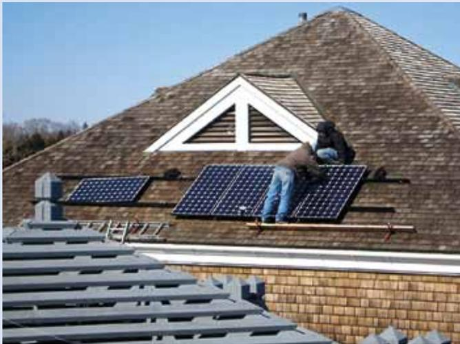
The Sandy Hook Foundation provided funding to install solar panels on the roof of the North Beach Plaza comfort station. The nine panels were installed by Sea Bright Solar in late February, each providing 230 watts during peak conditions. The power generated supplemented power needs at the comfort station during the main visitor season and will feed back to the utility company for the duration of the closed season. A planned
