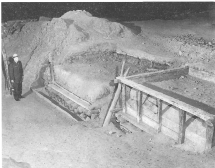
Fig. 13. Portion of the salt-peter mining operations which was carried on in Mammoth Cave during the War of 1812. Vats were used in the leaching of nitrates from the dry cave earth. These and other features of the operation may be seen on the Historic Trip. Photo by W. Ray Scott, National Park Concessions, Inc.
