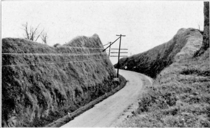
Figure 3.—Old Jackson Road cut into the Loess at the line of the Confederate trenches in the Vicksburg National Military Park. Although the verticality of the walls of the cut has been modified by recent improvement, nevertheless, the depth of the cut and the steepness of the walls are shown in this photograph of December 24, 1934.
