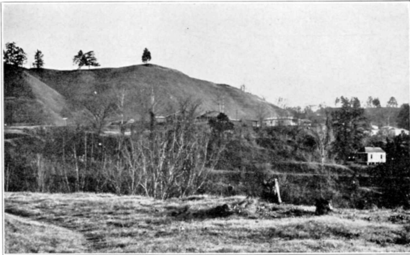
Figure 4.—Fort Hill across Mint Spring Falls from the National Cemetery.—This photograph of December 24, 1934 was taken shortly after the extremely steep bluff had been terraced and sodded.
