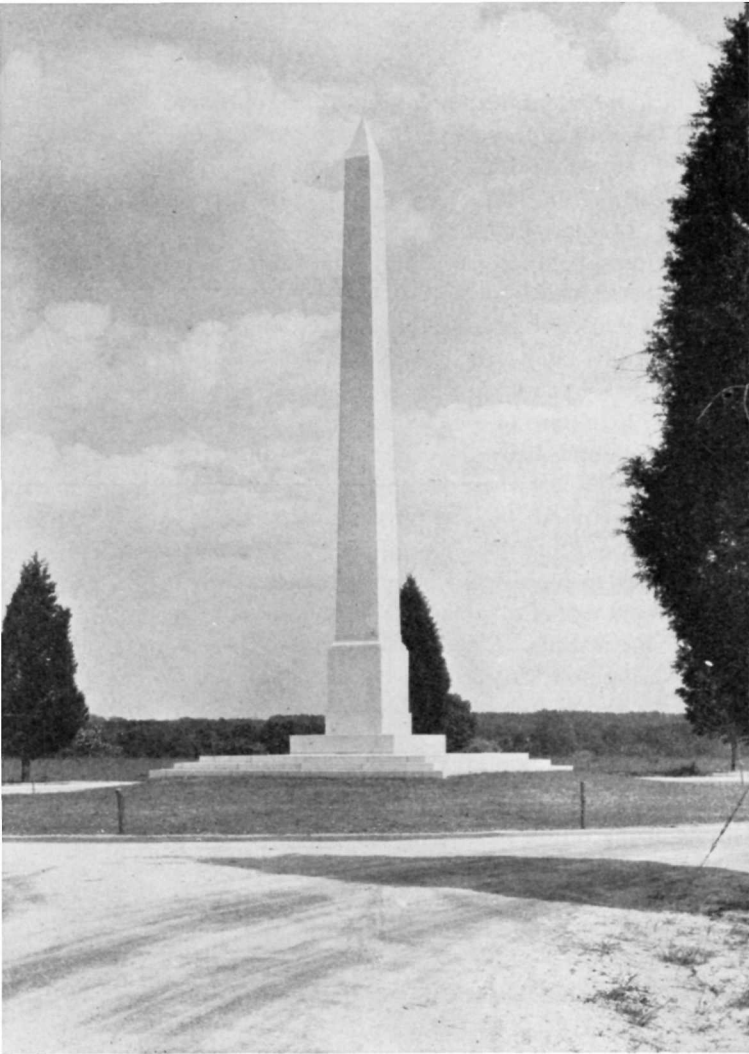
This shaft of Vermont granite weighing about 50 tons and nearly one-tenth the size of the Washington Monument in the Nation's Capital, and of the same relative proportions, was first erected in 1896 by the Federal Government on the site now occupied by the memorial mansion. In 1930 it was moved to its present location where it is encircled by the entrance road near the western boundary of the birthplace reservation
