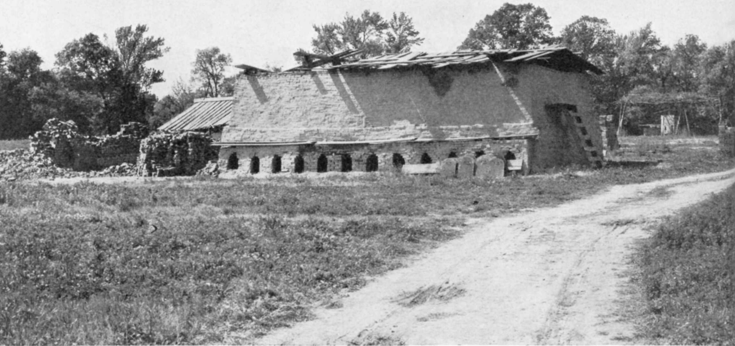
The brick used in constructing the memorial mansion were hand-made from clay taken from a pit near the house site and were burned in an old-fashioned up-draft Dutch kiln fired by oak and chestnut cordwood cut on the place
