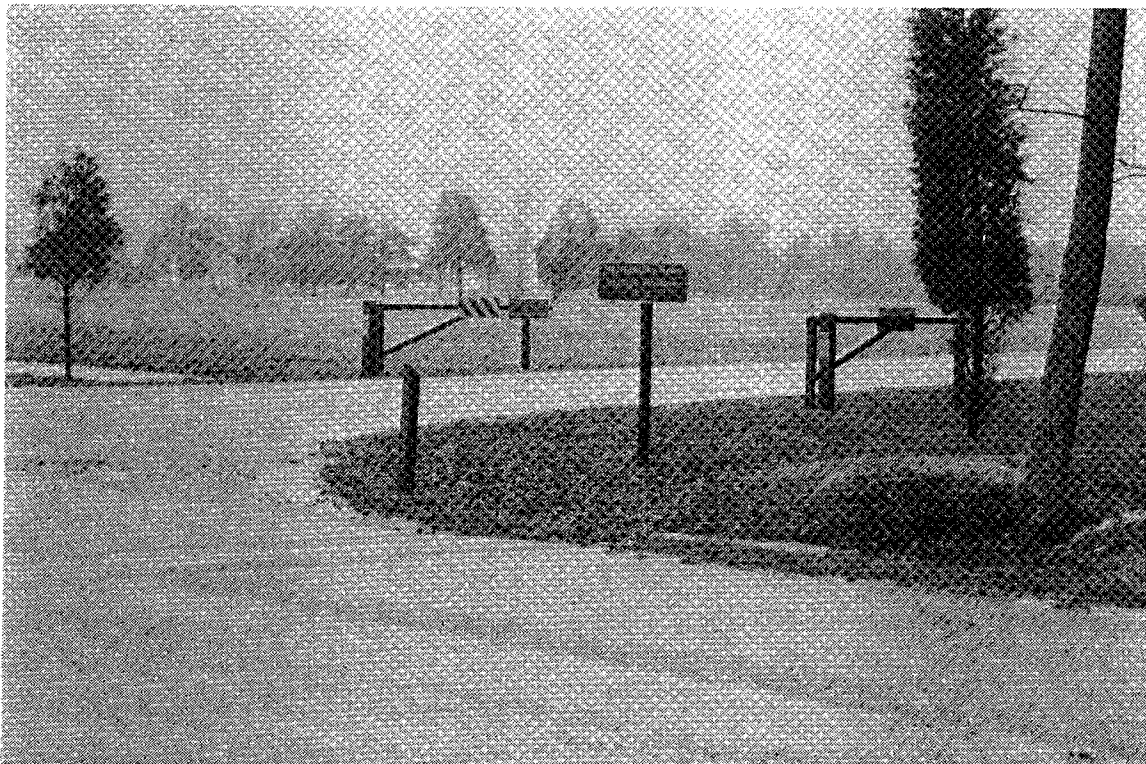
46. The access road to the maintenance area.
