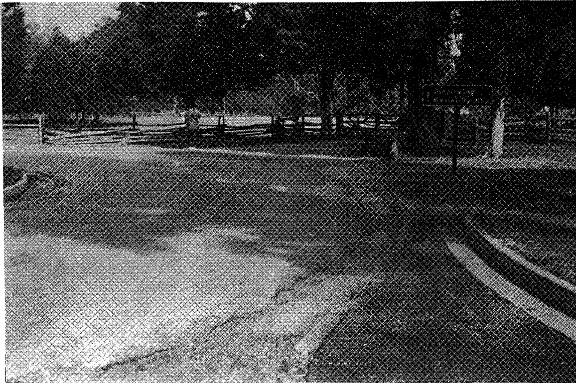
27. The traffic circle east of the monument. (See photo 11 in chapter 2 for a comparative view of historic conditions)
