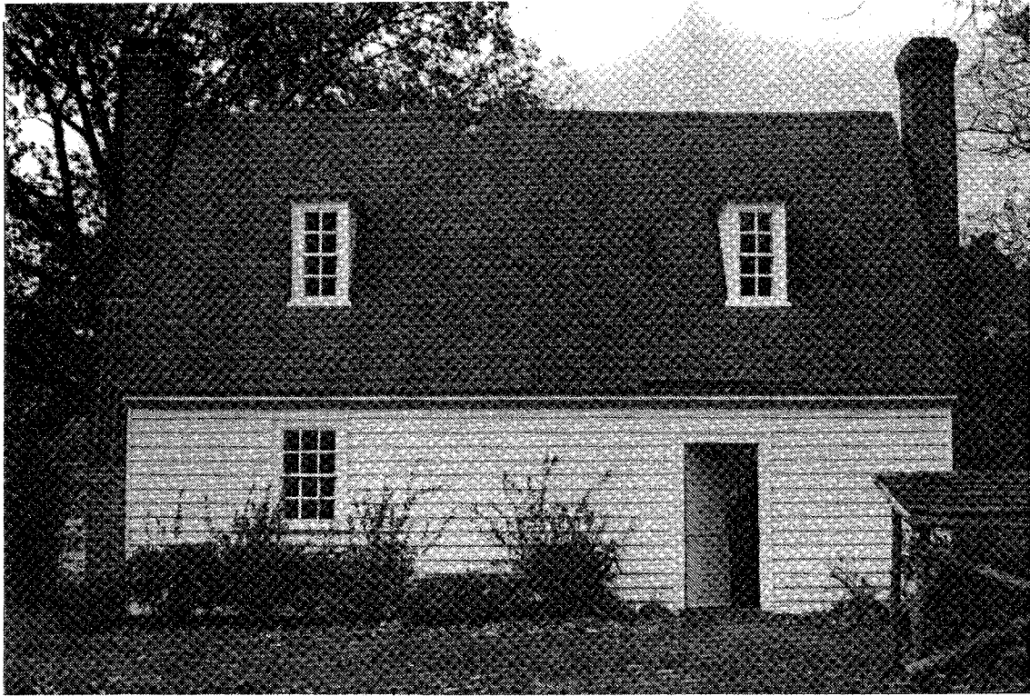
87. View northwest of the Kitchen House, also constructed in the 1930s. It is located 80 feet from the Memorial House. Costumed interpreters stationed here and elsewhere around the historic core provide visitors with information about eighteenth century life on the property.
