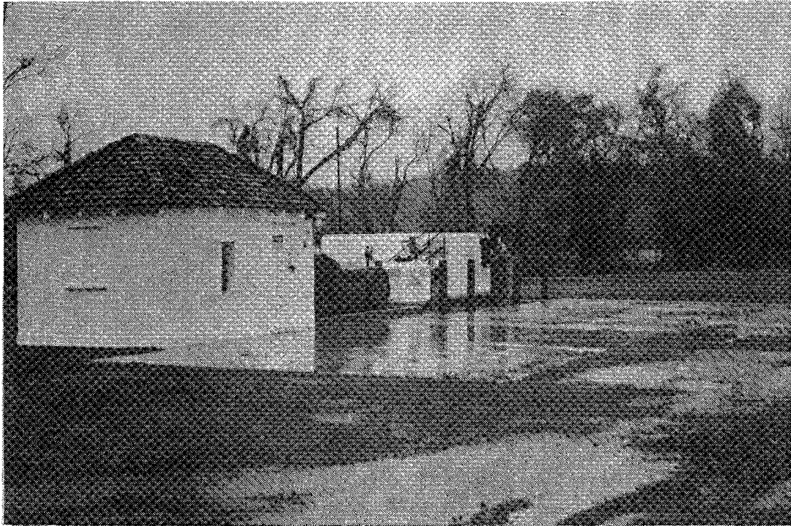
49. A cluster of utility structures are located in the maintenance area. The gas house provides fuel for maintenance vehicles.
