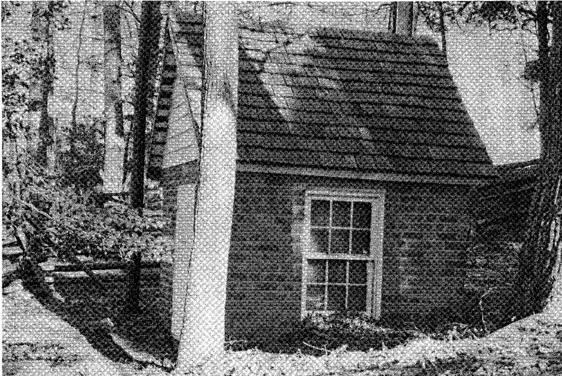
33. A brick pump house is located east of the Ice Pond and provides water to the historic core area.
