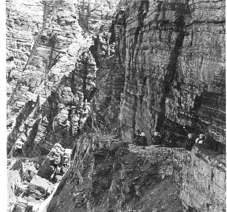
The trail on the north side of Ptarmigan Tunnel.
