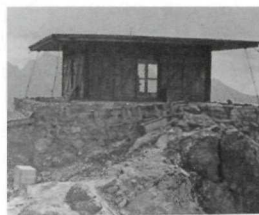
Construction of Heavens Peak Lookout
