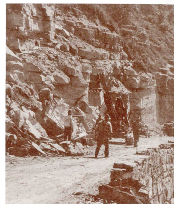
Contractors saved rock removed during excavation for use in masonry work. Sometimes they needed more rock, so they set up several quarries along the road. One quarry that was used extensively was just west of Haystack Creek.
