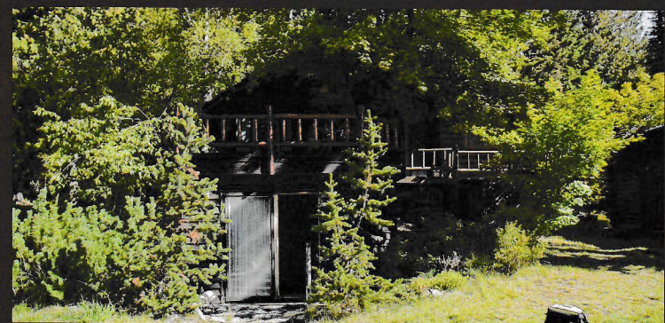
Left: Entrance to the Main Cabin
