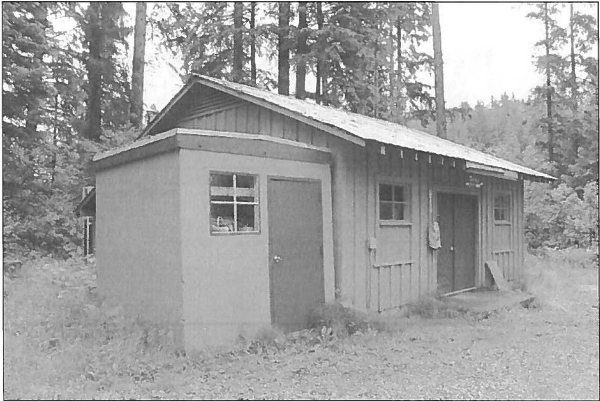
Photo 13: GBA-10 Recreation Center and Storage. Northeast and Northwest Elevations, facing south.
