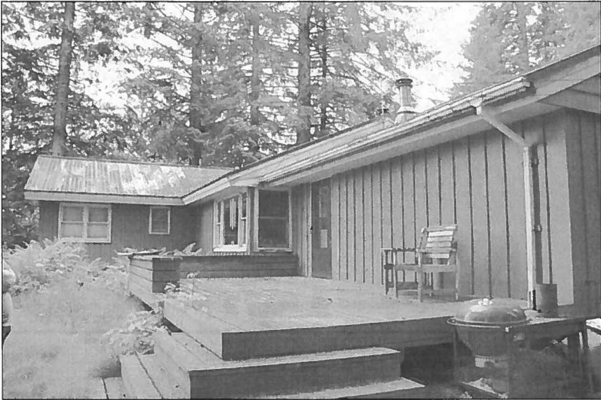
Photo 4: GBQ-5 Residence, Northeast Elevation facing southwest.
