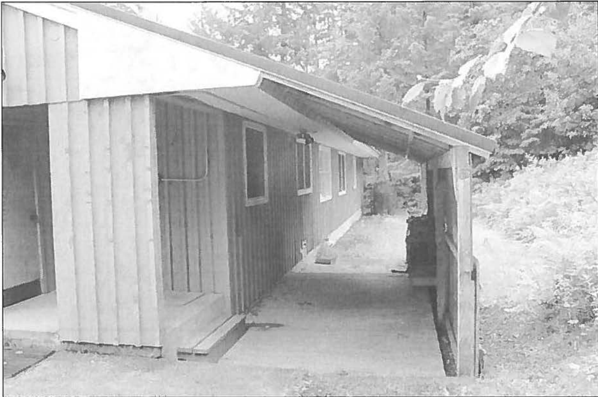
Photo 10: Building GBQ-3 Residence, South Elevation facing northeast.
