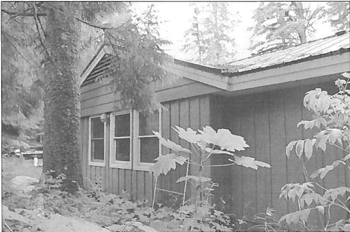
Photo 6: GBQ-5 Residence, Northeast Elevation facing southwest.
