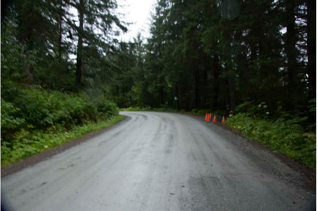
Photo 3: Administrative Road, Toward Southwest, Cones denotes Electrical Pull Box 13 location, NPS CLI program, 2017
