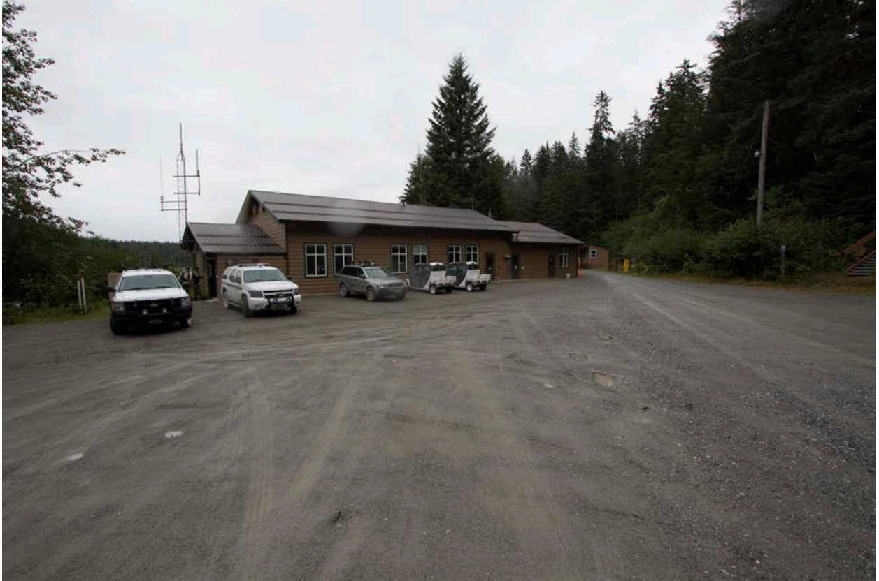
Photo 5: Headquarters Parking Area, Former Maintenance Building (now Resource Management Office) in background, Toward North, NPS CLI program, 2017
