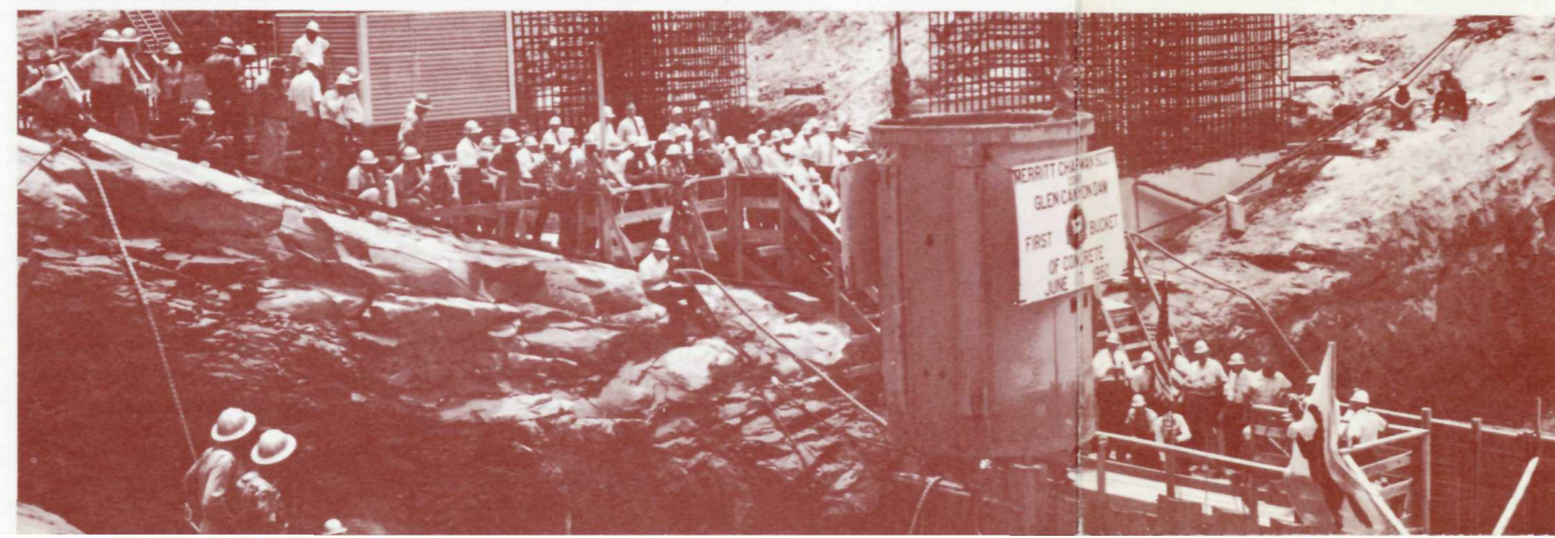
The first placement of concrete—June 17, 1960.
