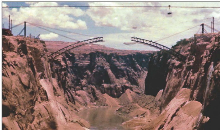
Colorado River Bridge construction, February, 1958
