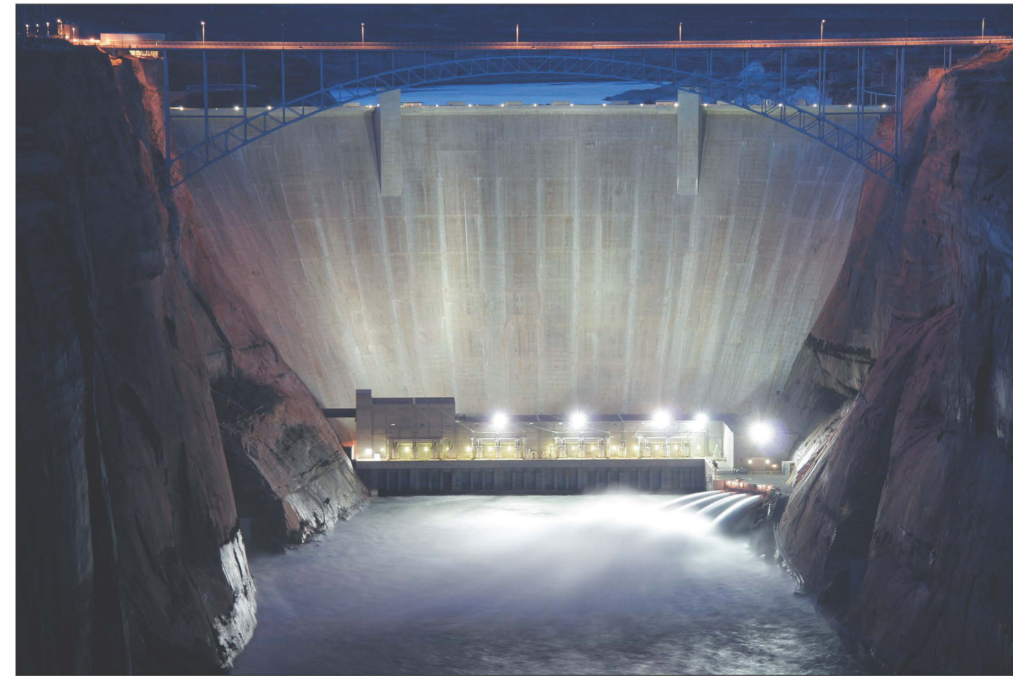
Night view of jet tubes during the March 2008 high-flow test
