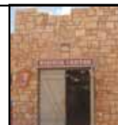
Navajo Bridge IC
