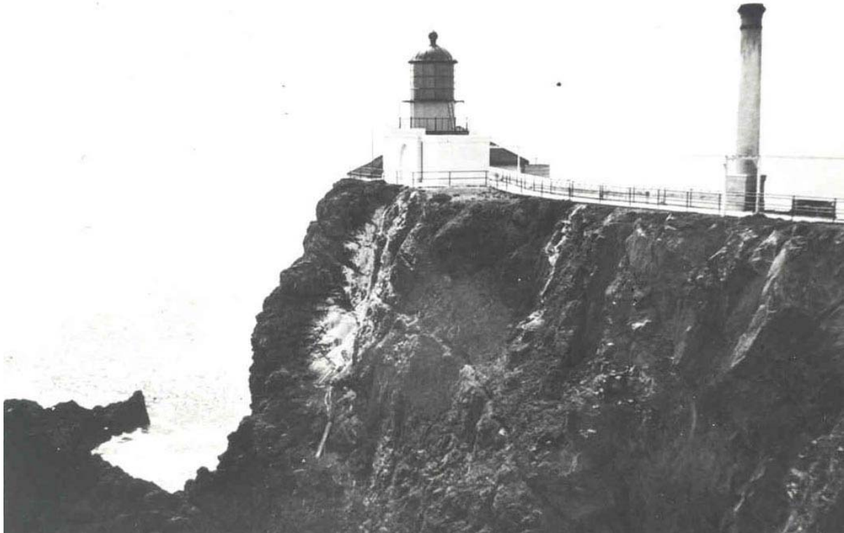
History #3: Circa 1910 view of the 1877 brick lighthouse, with the 1855 metal lantern and lamp rooms. The 1903 fog-signal building roof is in the background. The brick chimney for the fog-signal boilers is on the right. (U.S. Coast Guard, 12th District)
