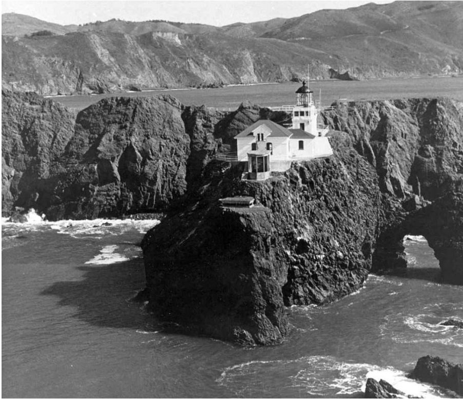
History #6: 1967 oblique aerial view (looking east) of the abandoned U.S. Army fire control station and searchlight enclosure in front of the 1903 fog-signal building and lighthouse tower. (U.S. Coast Guard, 12th District)
