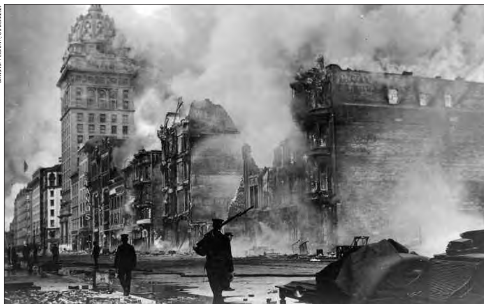
Looking east on Market Street, late morning, April 18, 1906, as the Call Building (tall structure at left of photo) burns. The fire started at the top, and as the heat became more intense, windows blew out. By afternoon, the building stood in ruins.
