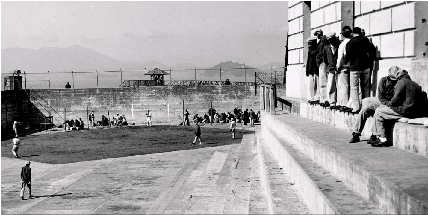
Inmates take advantage of a sunny 1940s day in the recreation yard; under the watchful eyes of the tower guards, the men converse, play baseball, and engage in lively games of bridge behind the backstop, sheltered from the wind by the yard's high concrete walls.
