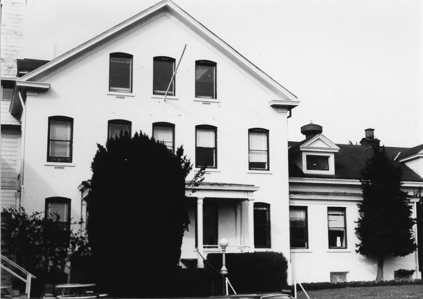
1. Brick portion of the headquarters building, San Francisco Port of Embarkation, Fort Mason. The U.S. Army constructed this unit as a posh hospital in 1902.
