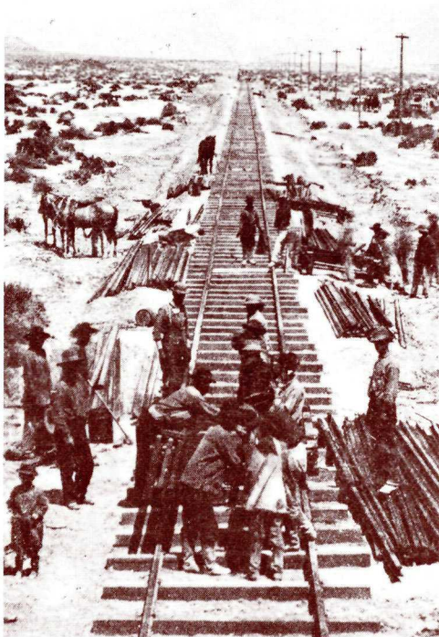
Railroad construction was labor intensive, with each worker assigned a specific job.
