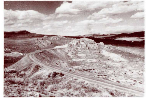
Central Pacific's "Big Fill" as it looks today.
