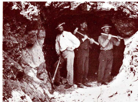
Drilling crew with the tools of their trade.
