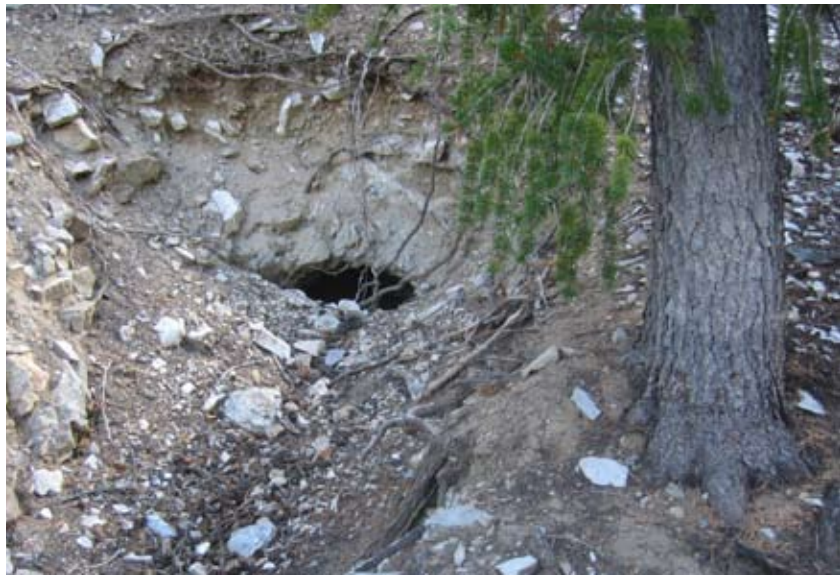
Figure 2. Partially collapsed mining adit in the backcountry.
