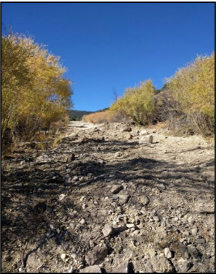
Road prior to road base removal
