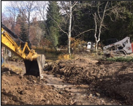
Recontouring streambanks after culvert removal
