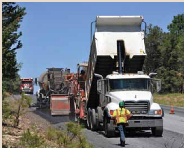
This pavement preservation project involved crack sealing, chip sealing, and restriping most of the paved roads on the North and South Rims of Grand Canyon National Park. This seal coat will provide seven or more years of service without the need to rebuild the sub base and resurface the asphalt.
