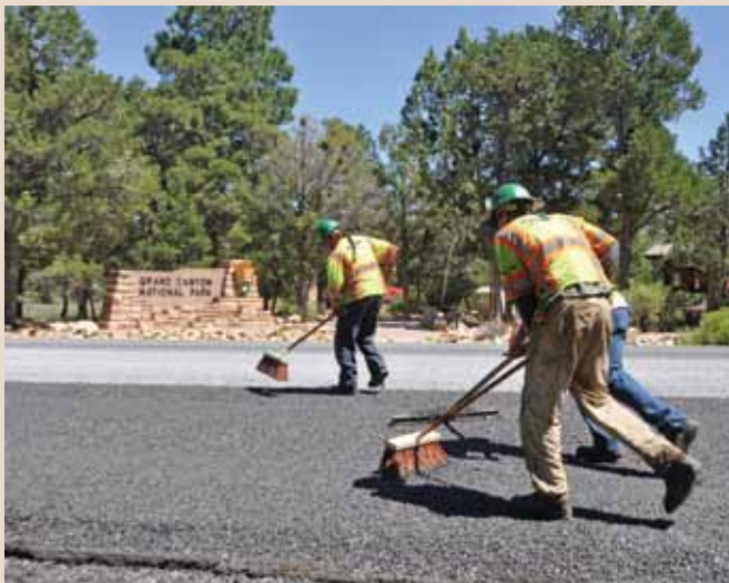
This pavement preservation project involved crack sealing, chip sealing, and restriping most of the paved roads on the North and South Rims of Grand Canyon National Park. This seal coat will provide seven or more years of service without the need to rebuild the sub base and resurface the asphalt.
