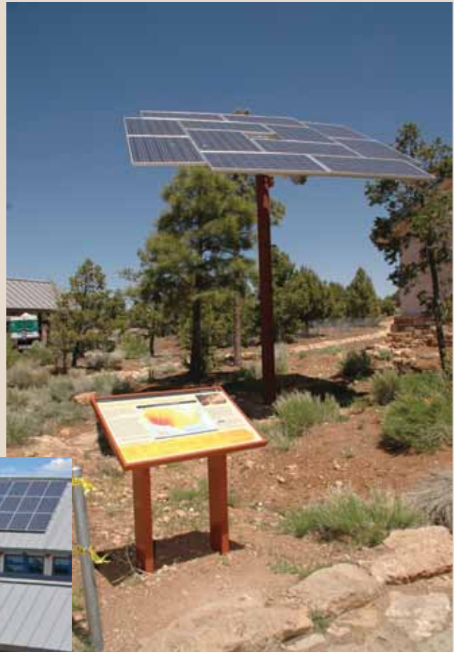
The Grand Canyon Visitor Center (South Rim), with the photovoltaic solar panels in place. The photovoltaic system is producing about 30 percent of the power used by the visitor center. NPS photos
