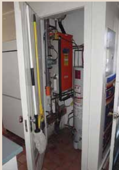
Improvements to the utility systems at Tuweep residence. NPS photo
