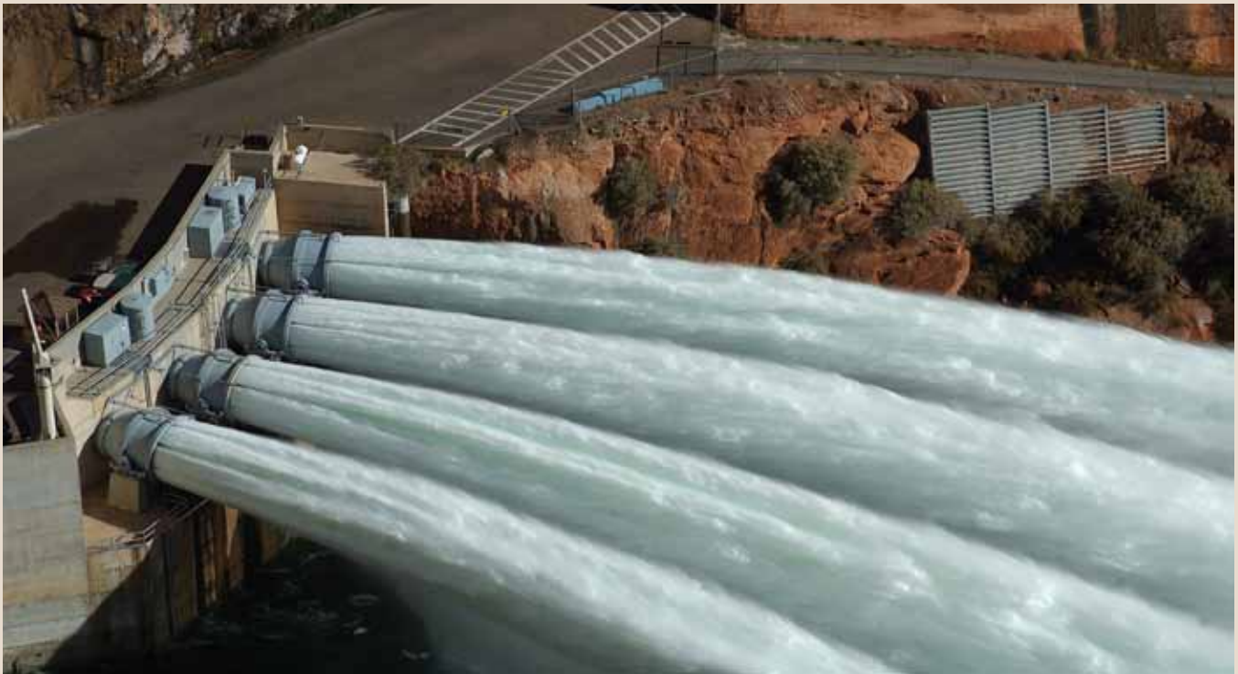
Water release from Glen Canyon Dam during a high-flow experiment. NPS photo
