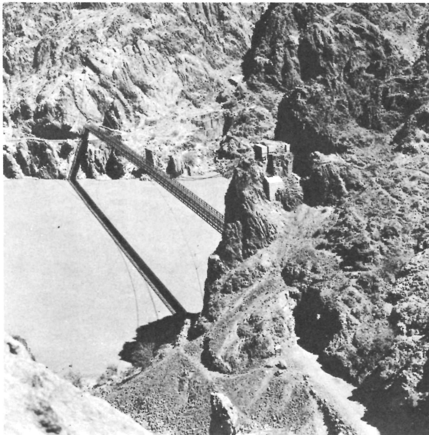
SUSPENSION BRIDGE OVER THE COLORADO
