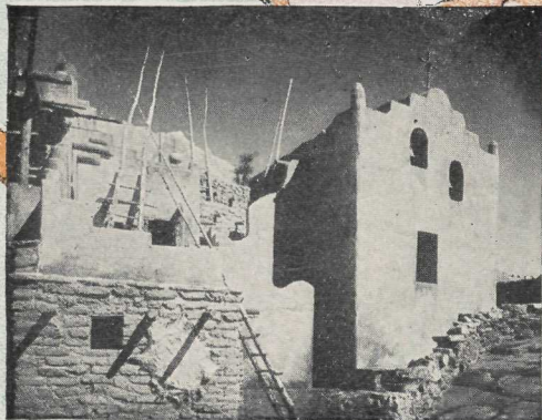
The Old Church and Part of Trail
