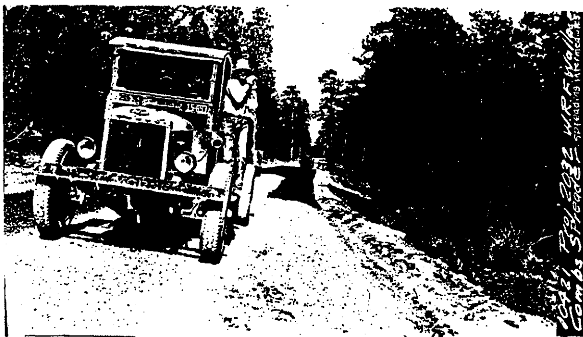
Figures 4 and 5. Subgrading (above) and surfacing (below) for 1927-28 South Entrance Road Construction. (Final Construction Report, GCNP Study Collection)
