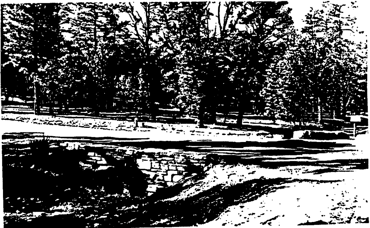
Figure 19. Headwall at southwest corner of Boulder Street and Center Road. The top of Boulder Street Headwall #1 is visible across the street. (From December 1936 Construction Report, GCNP Study Collection)
