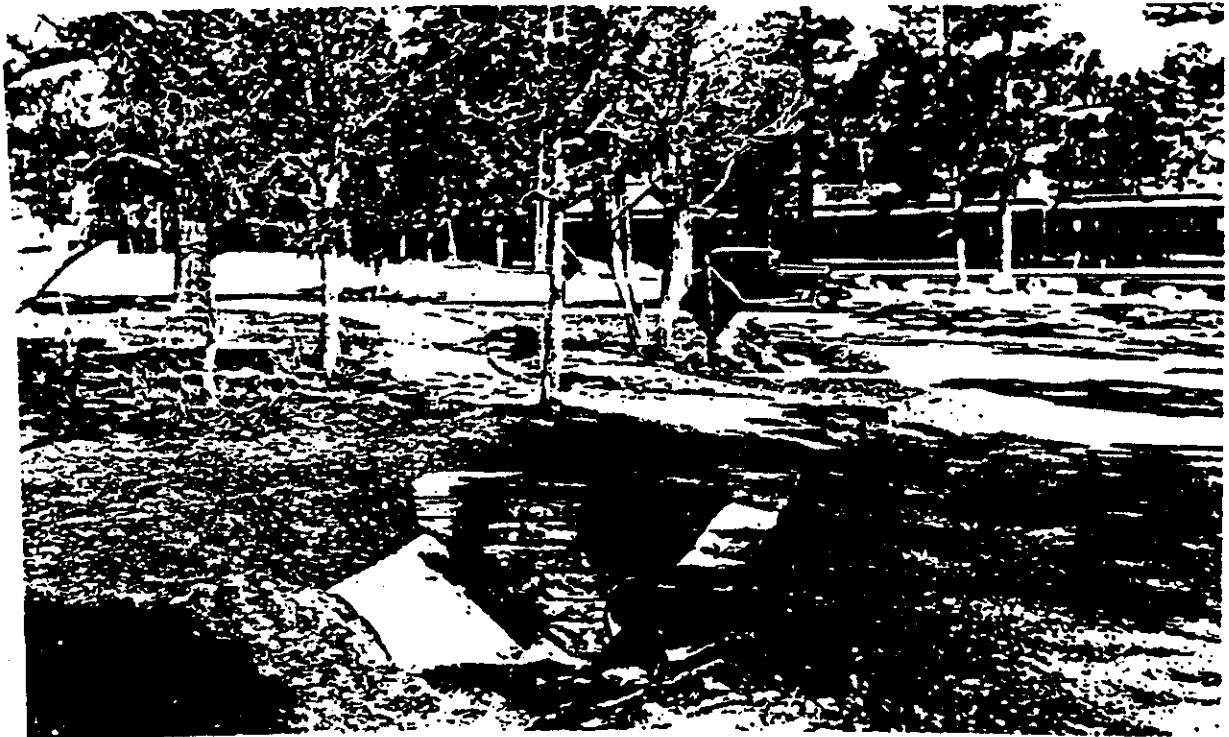
Figure 7. Apron, culvert, and headwall on Navajo Street built by C.W.A. crews between December 1933 and April 1934. Not all road structures were built by the C.C.C. (CCC reports, GCNP Study Collection)
