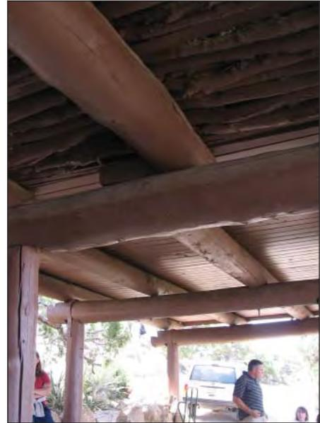
FIG. E22: View under the porch roof facing southwest showing the ceiling treatments of the historic porch at upper left and the addition roof at right, 2007.
