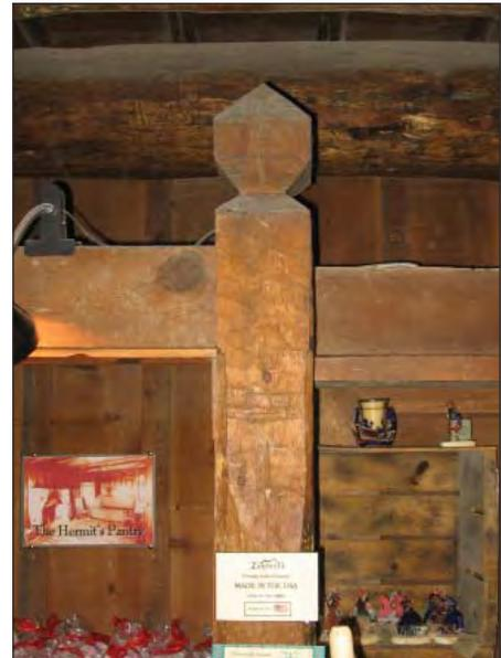
FIG. SR4: Detail of a finial on the south partition wall, 2007.
