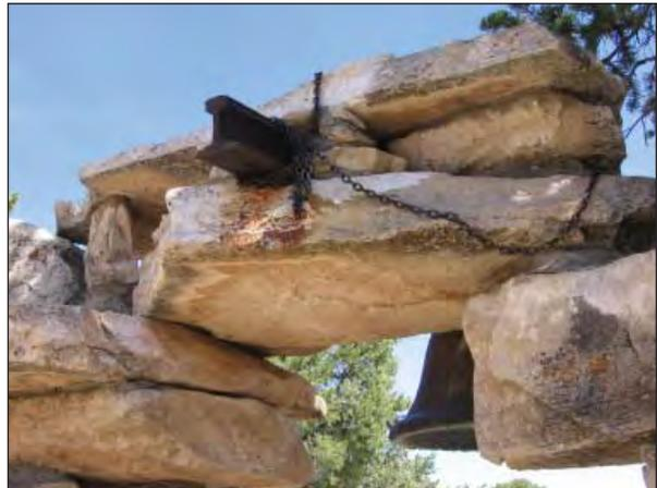
FIG. S31: Railroad track support for the bell on the corbel arch, 2007.
