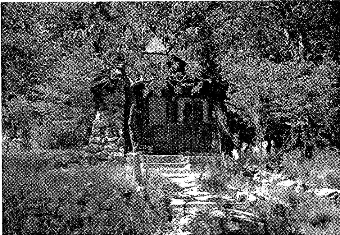
*Figure 7. The image illustrates the principal elevation of the Trail Caretaker's Residence at Indian Garden. From this angle, the aesthetic effects of the 1960 alteration and removal of the stone corner pier from the main facade are most noticeable, changing the balance and symmetry of the composition. Note the prominence of the role of landscaping to the project. ARG Photo dated May, 2000.*
