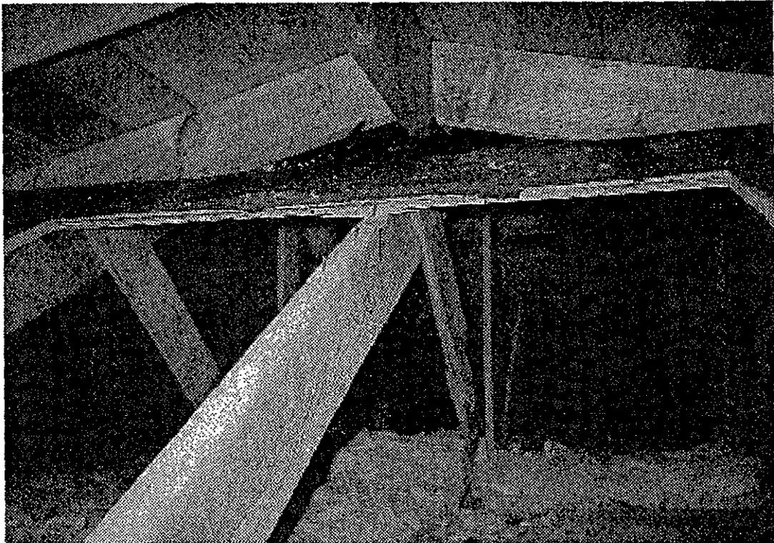
*Figure 12. The image illustrates the cabin's interior roof framing showing the original part of the structure in the rear and the newer truss construction completed in 1960. ARG Photo dated May, 2000.*
