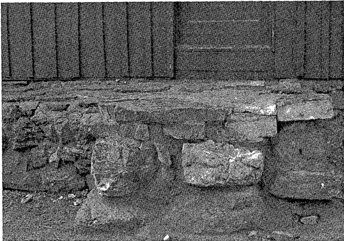
*Figure 6. The photo is taken of the stone porch that runs along the west elevation of the Trail Caretaker's Residence and below the door added in the 1960 works. It is thought that the porch and other elements of the 1960 alteration re-use stones that were dismantled from two of the four original corner piers. ARG Photo dated May, 2000.*
