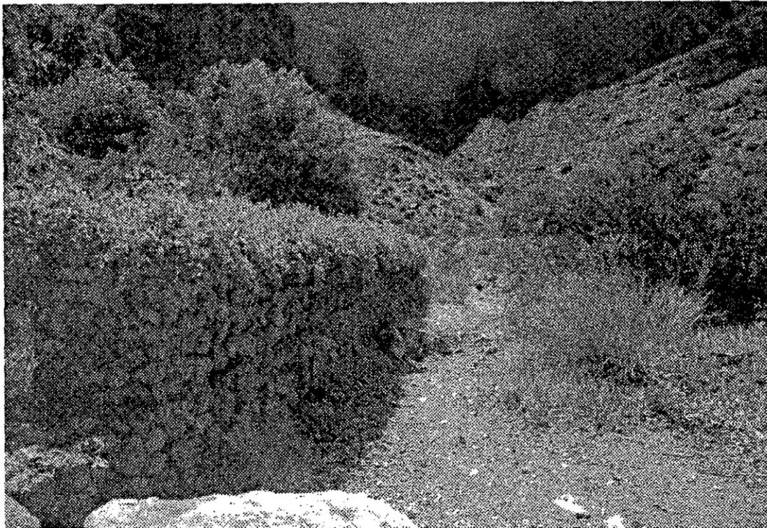
*Figure 3. The image illustrates the gabion walls that mark the southern boundary of the immediate environs of the Trail Caretaker's Residence at Indian Garden. The rock walls measure approximately 5' in height and are constructed like a wire cage filled with stones to divert run-off and act to prevent damage during flooding. View is looking southwest from behind the structures. ARG Photo dated May, 2000.*
