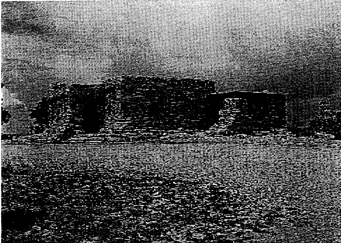
Figure 16. - The image shows view of the east elevation of the Yavapai Observation Station from the southeast. GCNPA Photo Number 9750. Photo dated July, 1930 by George Grant.
