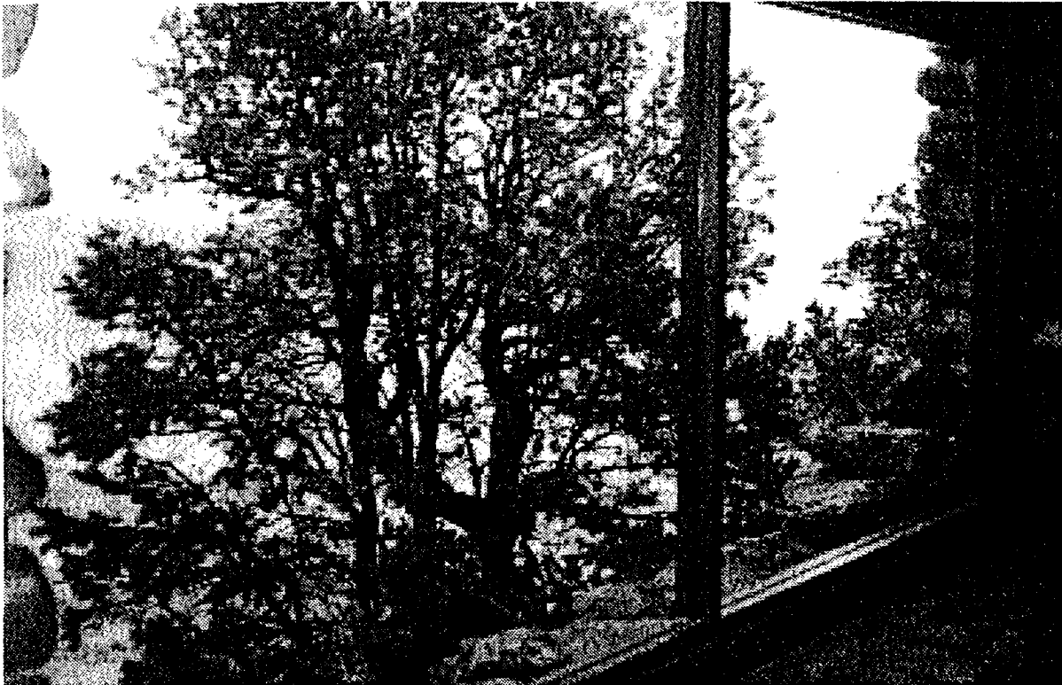
Figure 18. This image illustrates the windows on the east side of the Yavapai interior, inside the foyer entrance. The windows were installed in 1979, replacing the 1953 glazing. The windows look to the north. Photo dated May, 2000.
