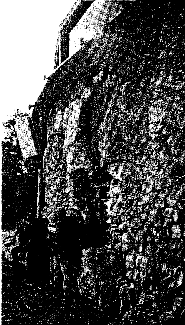
Figure 8. This image illustrates the lower northern side of the Yavapai exterior. Photo dated March, 2000.
