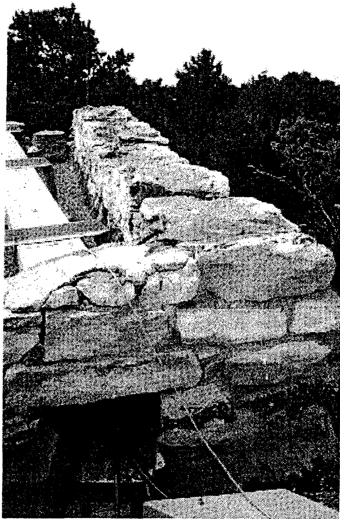
Figure 19. This image illustrates the parapet above the flat roof. Evidence of mastic repairs. View is looking south. Photo dated May, 2000.
