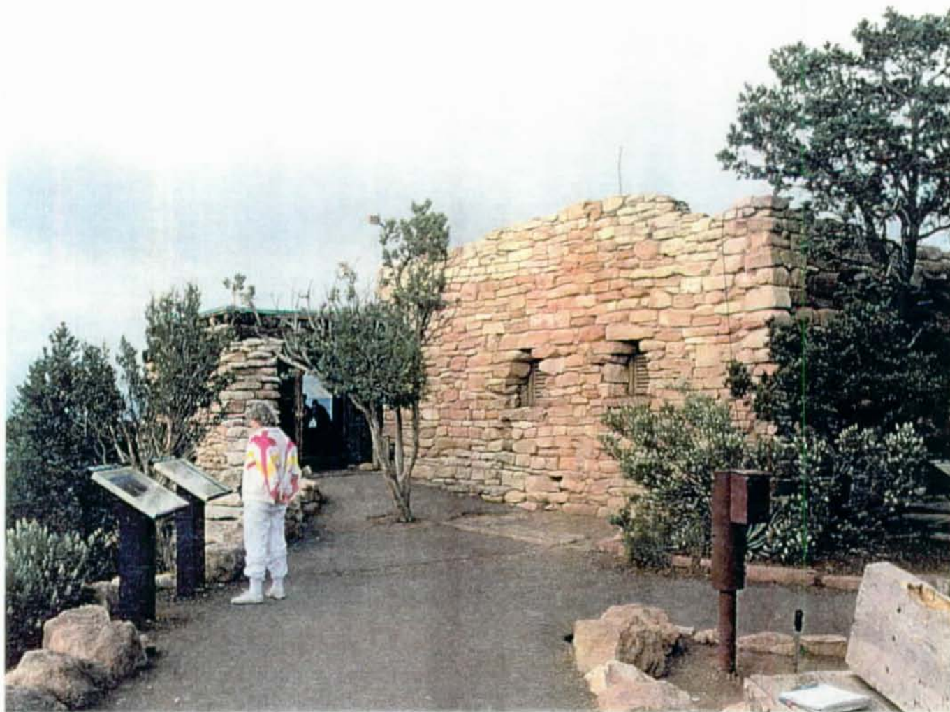
ELEVATION LOOKING NORTHEAST
