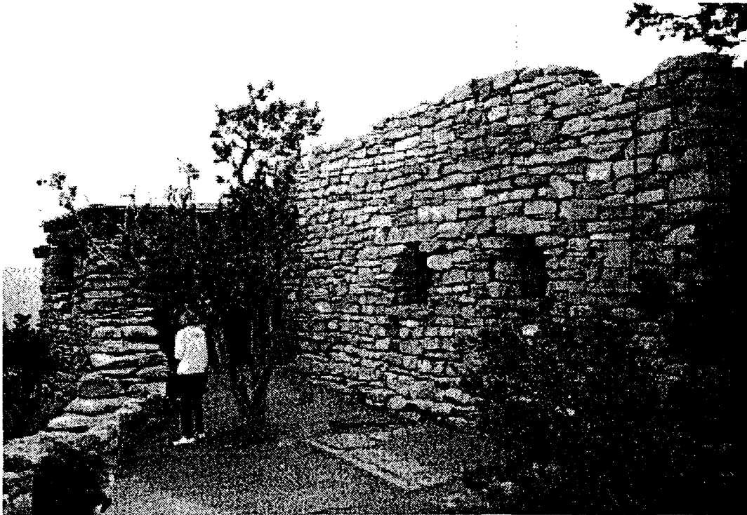
Figure 4. This image illustrates the west side of the Yavapai building. Photo dated May, 2000.
