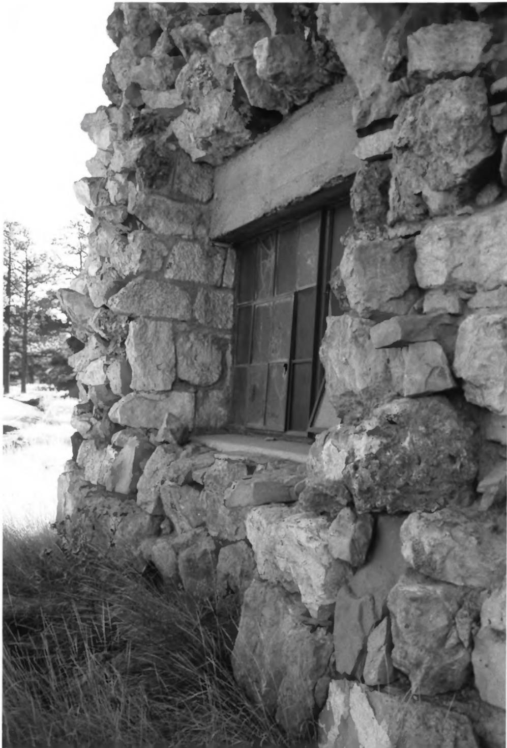
Corner of power house showing stone and concrete work and steel-sash industrial windows.
