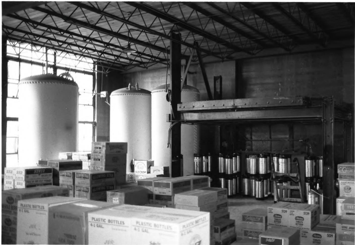
Grand Canyon Power House interior. Tanks and heavy steel work on the right are original. Space framing and wood decking above are recent additions, but are totally removable and are not attached to the structure.
