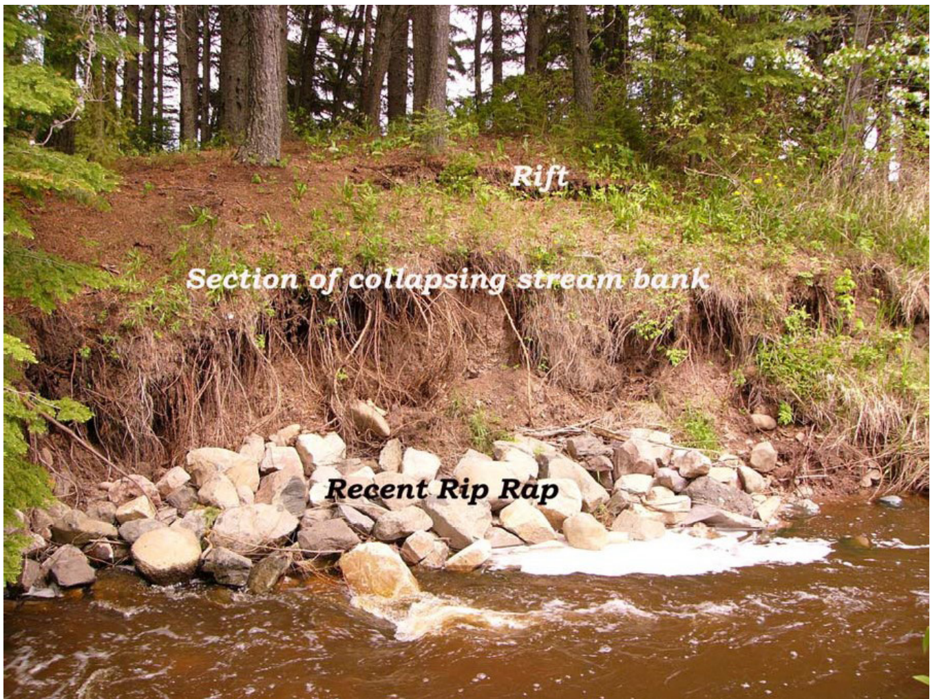
Figure 12. Photograph of a meandering section of Grand Portage Creek. Riprap was installed prior to 2005 in an attempt to stabilize the bank and prevent loss of cultural resources. View is to the east, just below the old ford, upstream of the stone bridge. Annotated graphic is figure 12 in Birk (2006).
