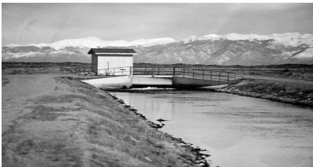
**Figure 3** View of Parshall Flume & Conveyance Channel
